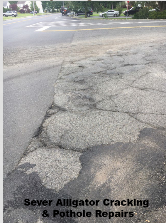
Sever Alligator Cracking & Pothole Repairs
