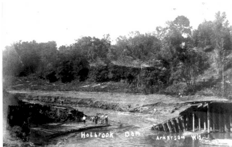
These are the remains of the Holbrook Dam.
