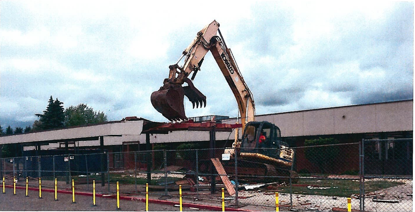
HIGH SCHOOL – Demolition underway for front canopy
