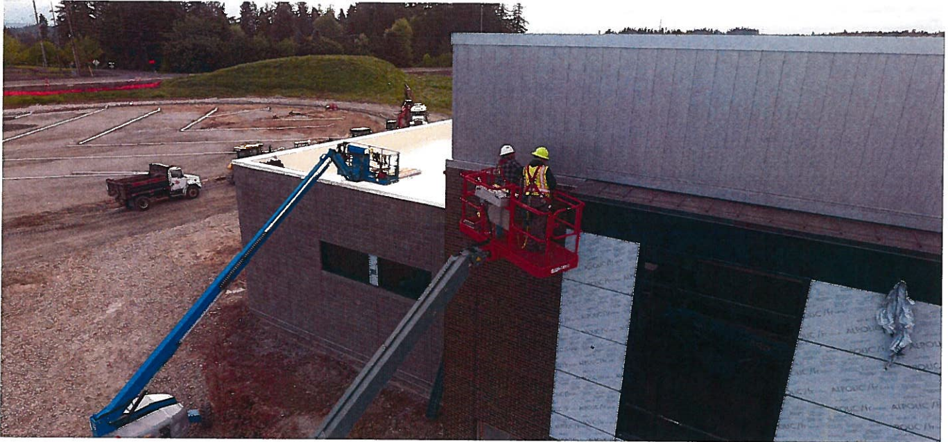
MIDDLE SCHOOL – Applying gym siding
