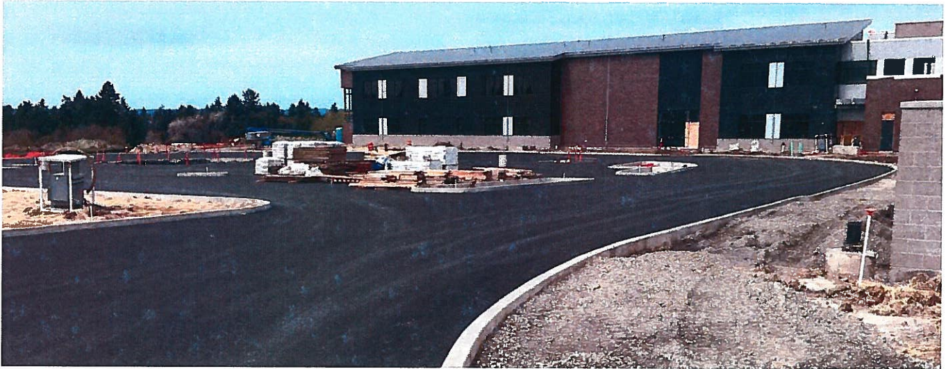
South (rear) lot is paved.
