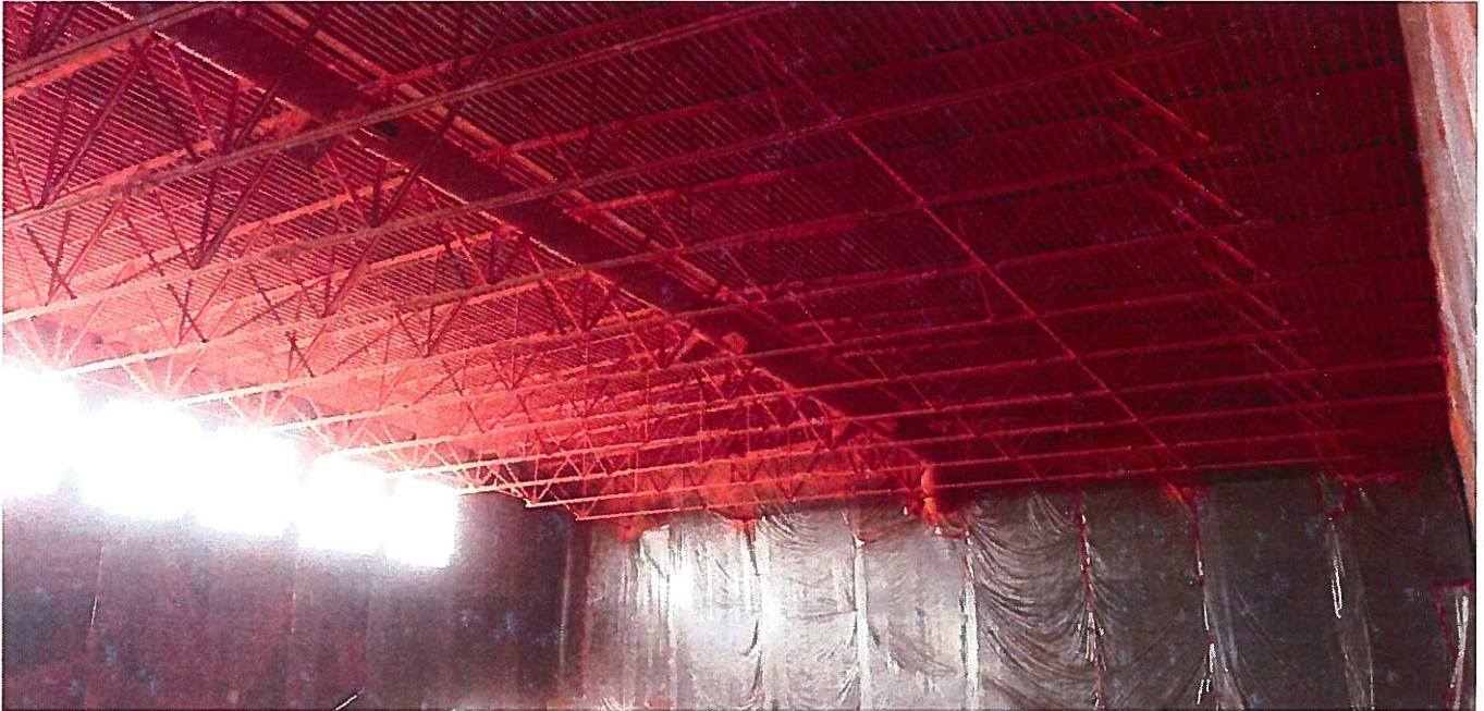
Main gym roof deck getting painted Ridgefield orange.
