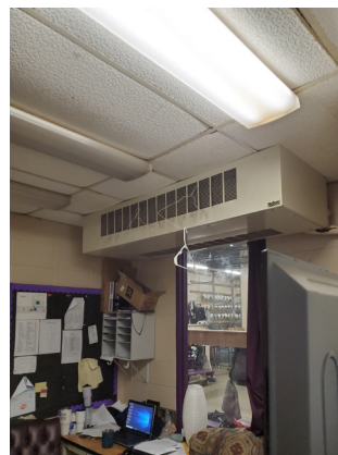
16.10 - Unit ventilators pose noise constraints
