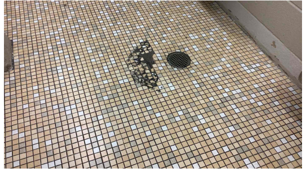
9.1b - Bathroom mosaic tile cracked and missing in locations
