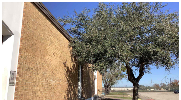
2.4b - Trees and bushes along building need to be trimmed to prevent damage to walls, roof, flashing or other building components
