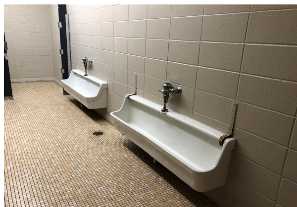
16.14 - Trough urinals are not ADA/TAS compliant
