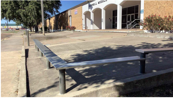
1.13 - Main entrance elevated with no ramp and steep grade between stairs
