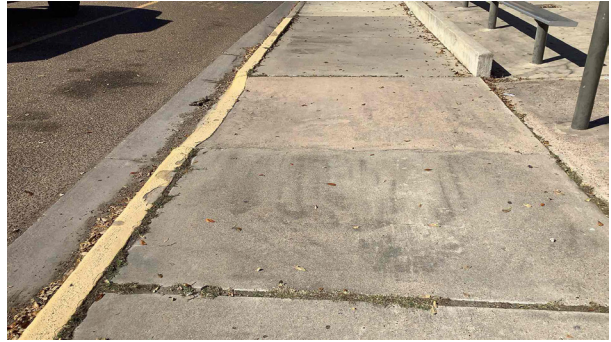
1.20 - Curb ramp flares create cross slope greater than 2%
