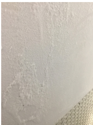
15.1c - Walk-in cooler freezer - frost build-up on freezer door
