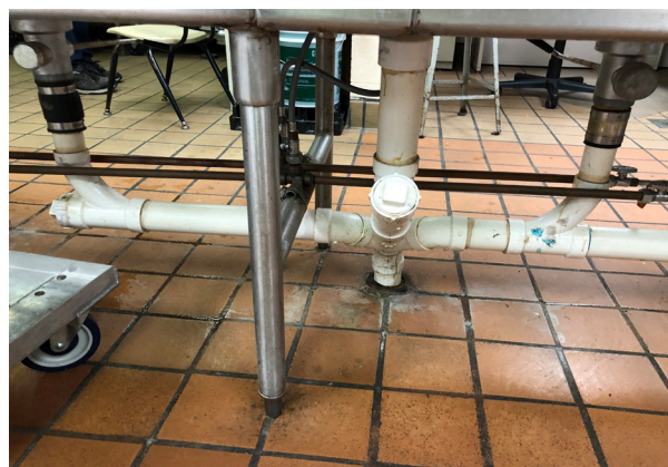
16.12 - Plumbing 3 compartment sink drain (MEP) must discharge into floor drain
