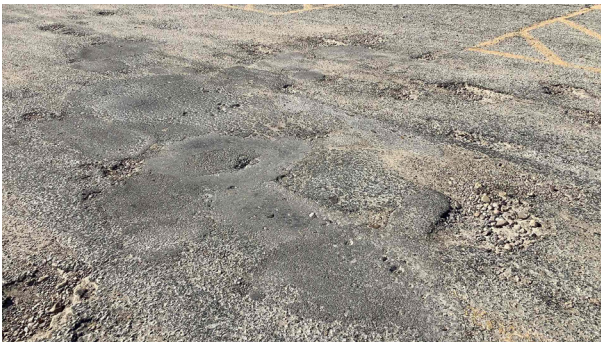
3.3b - Heavily deteriorated and potholed staff parking lot
