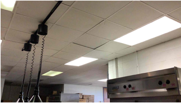
15.6 - Ceiling tile dirty, ceiling grid sagging and missing tile
