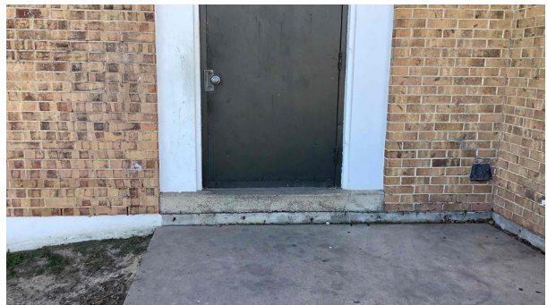
5.4 - Locations where concrete is settling adjacent to building creating step hazards and exposing concrete dowels
