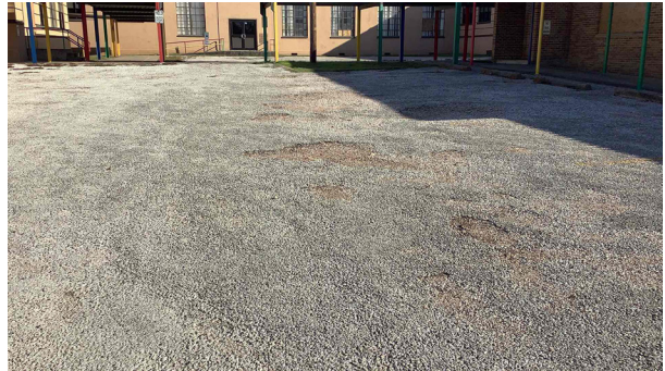
3.3a - Heavily deteriorated and potholed staff parking lot
