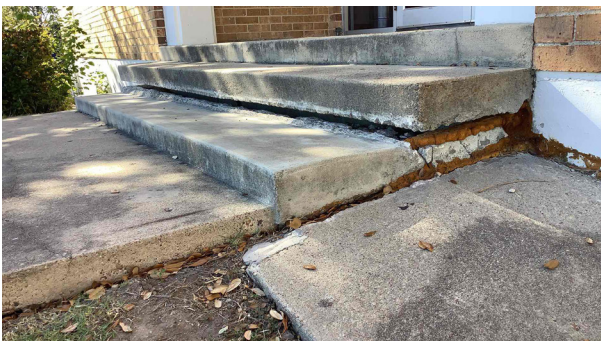
5.5a - Concrete walk at main and side entrances settling creating "floating" step – not compliant with code for step heights and concern step could break/ collapse
