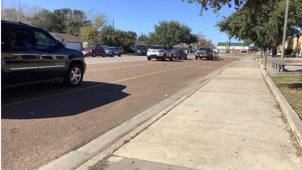
3.1 - No accessible pedestrian loading zone along drop off/ pickup area; multiple lanes for pickup causing students to walk across lanes of traffic
