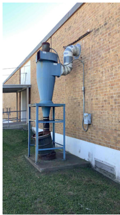
16.1 - Exterior dust collection barrel rusted – evidence that roof cover for dust collector removed
