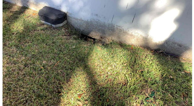
2.2 - Erosion along building edge exposing building underfloor allowing access for water and critters under building
