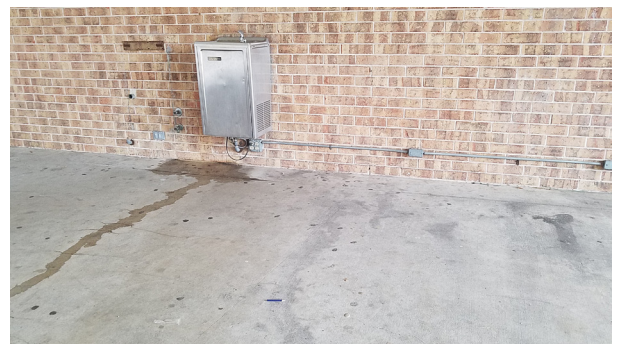
16.4 - Exposed non-GFCI electrical outlets at non compliant drinking fountain (exterior, wet area)
