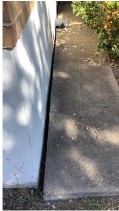
5.3 - Concrete mow strip along building edge pulling away with no concrete sealant
