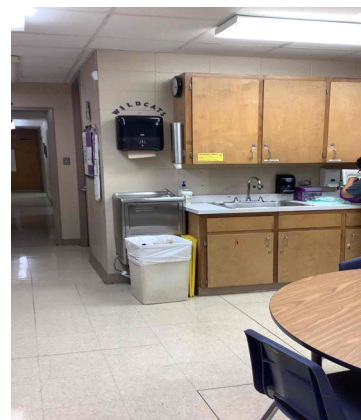
12.2 - Sink base cabinets not compliant for accessibility
