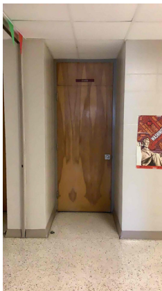
1.5 - Inadequate clearance on pull side of door
