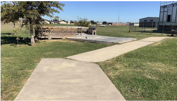
1.9 - Concrete path is disjointed with tripping hazard
