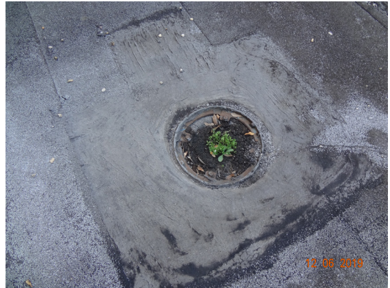
Roof drain strainer missing and drain body filled with debris and growing plants
