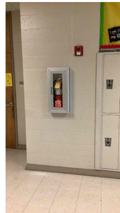
1.10 - Fire extinguisher cabinet mounted too high – handle above 48 inches
