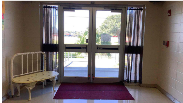
10.1 - Bottom rail of existing storefront doors (must be 10" for accessibility)
