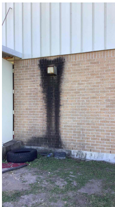
6.5 - Growth of exterior walls (potential cavity ventilation issue)
