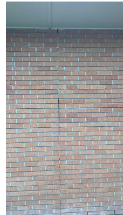
6.4 - Building sealants drying out, cracking and failing allowing moisture into building envelope
