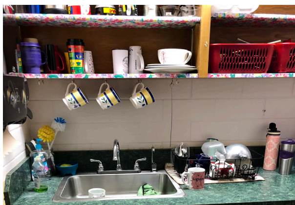
16.13 - No knee clearance provided below sink
