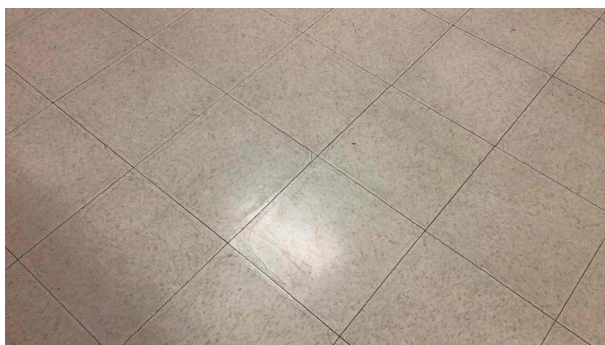
9.7b - VCT gaps (likely due to movement of tile from adhesive failure)
