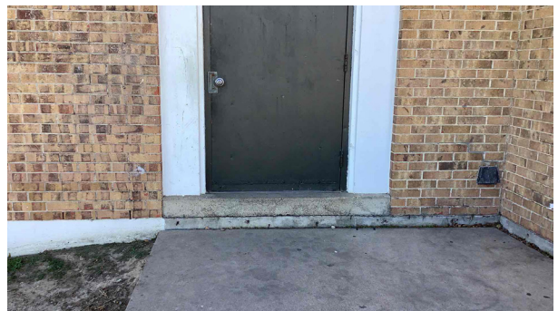
1.6 - No landing or ramp at exterior door step for access
