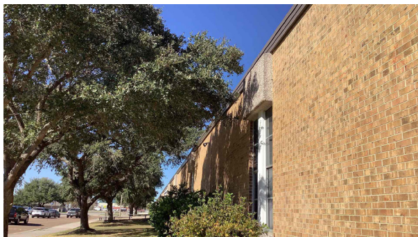
2.4a - Trees and bushes along building need to be trimmed to prevent damage to walls, roof, flashing or other building components
