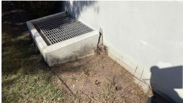
4.1 - Areaway attachment to building broken causing areaway to shift
