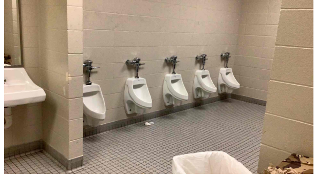
1.2 - Bathrooms (fixtures, partitions, mirror reflective surface height, trap insulation). Bathrooms with 6 or more fixtures have both accessible and ambulatory toilet stall
