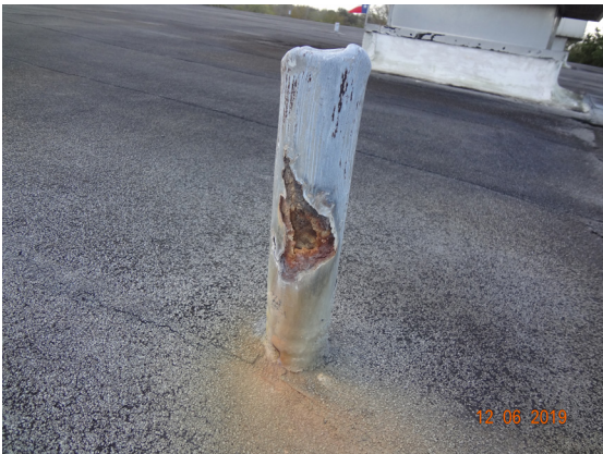
Damaged and rusted lead flashing was observed installed to vent pipe penetrations.
