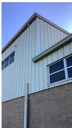
8.1 - Gutter downspouts disconnected from gutter at roof
