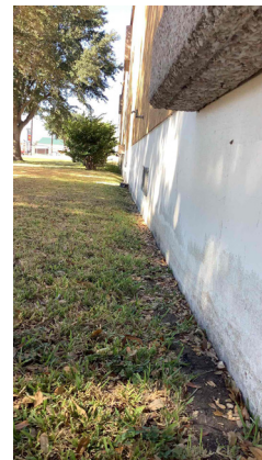
2.3b - Negative slope towards building prevents positive drainage away from building
