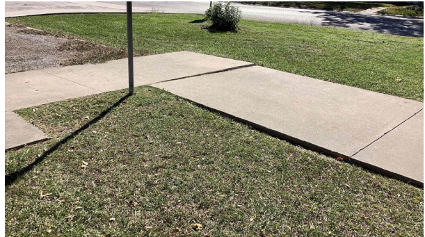
5.2 - Concrete walks heaving and moving - accessibility issues
