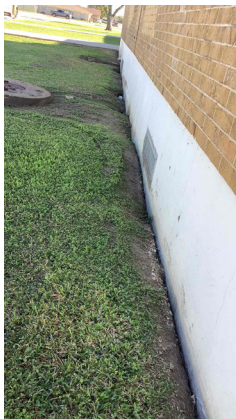
2.3a - Negative slope towards building prevents positive drainage away from building
