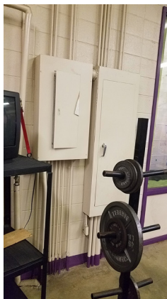
16.7 - Panels unlocked and accessible in weight room
