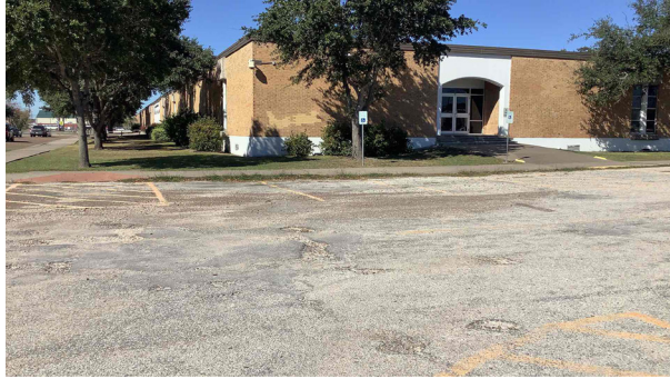
1.1 - Accessible parking not properly identified with signage, access aisles, and accessible route to sidewalk (potentially not sufficient accessible parking – verify counts)
