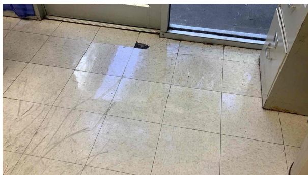
9.9 - VCT curling at corners and edges and damaged at exterior door (wet) location
