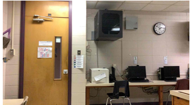
14.2 - No traditional MDF and IDF closets – cabinets located where possible
