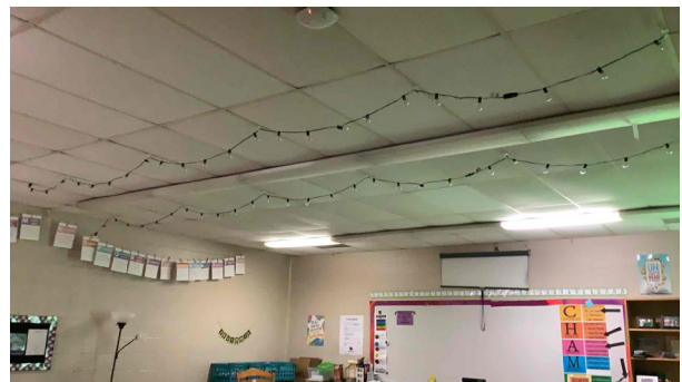
16.8c - Many interior light bulbs out in fluorescent fixtures
