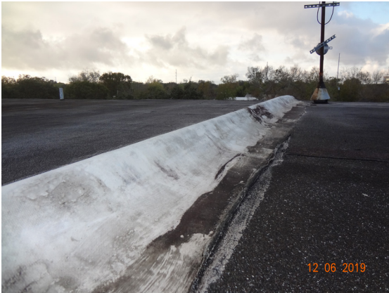
Materials installed to expansion joints appeared to be deteriorated and brittle
