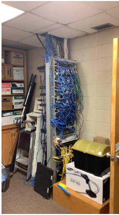
14.1 - No traditional MDF and IDF closets – cabinets located where possible
