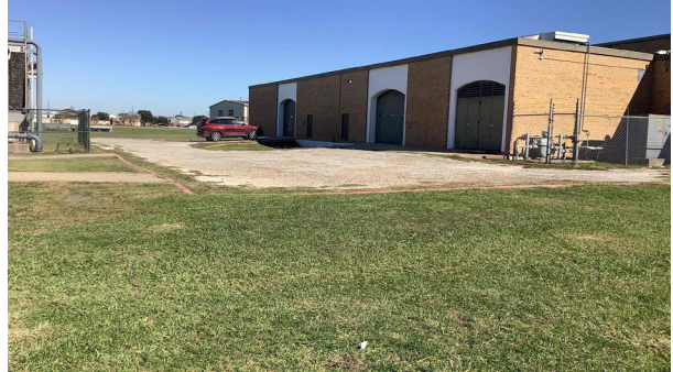
3.2a - Service drive/ fire lane severely potholed and deteriorated
