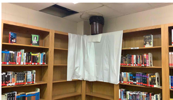
8.3b - Roof leak in library forcing removal of books and draping shelves with plastic
