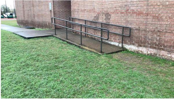
1.19 - Ramp to nowhere block ramp at landing or extend walk beyond
