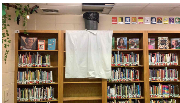
8.3a - Roof leak in library forcing removal of books and draping shelves with plastic
