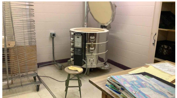
9.3 - Kiln sitting directly on VCT – should be on concrete or similar
