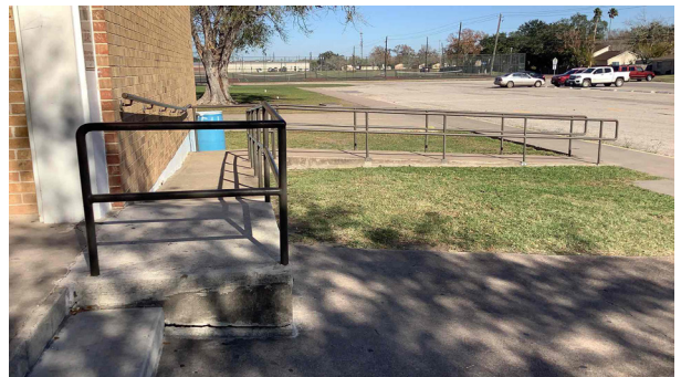
1.18 - Ramp handrails not compliant and stairs missing handrails
