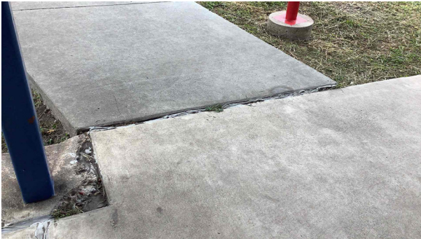
5.1 - Concrete settling at step allowing water under flatwork
