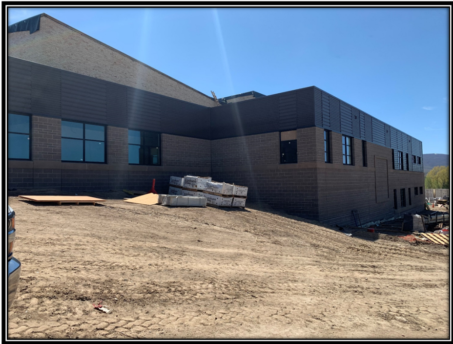
Photo taken on 5/5/20, building exterior, east elevation. Masonry & metal panel work is complete in this area.
