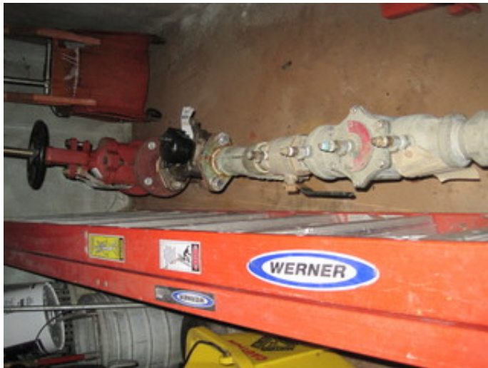
Water meter & backflow preventer
