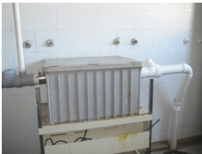
Kitchen grease waste interceptor
