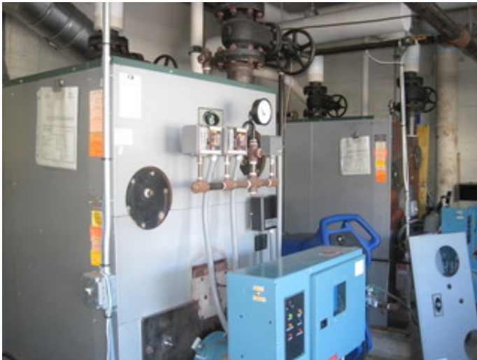
Steam heating boilers
