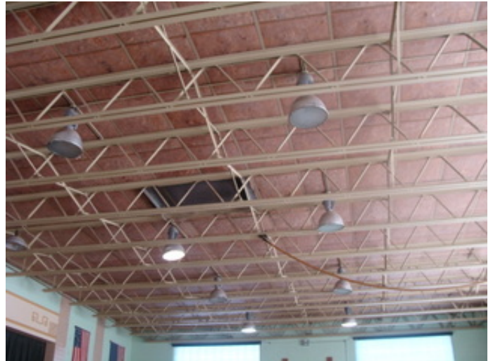
Steel Trusses at Gym
