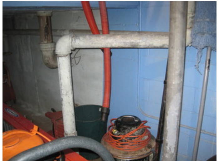
Galvanized domestic water piping
