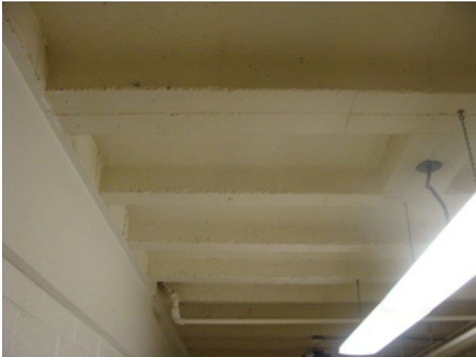
Poured Slab above basement floor
