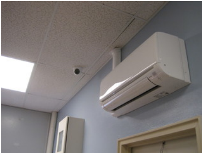
Ductless split-system A/C unit
