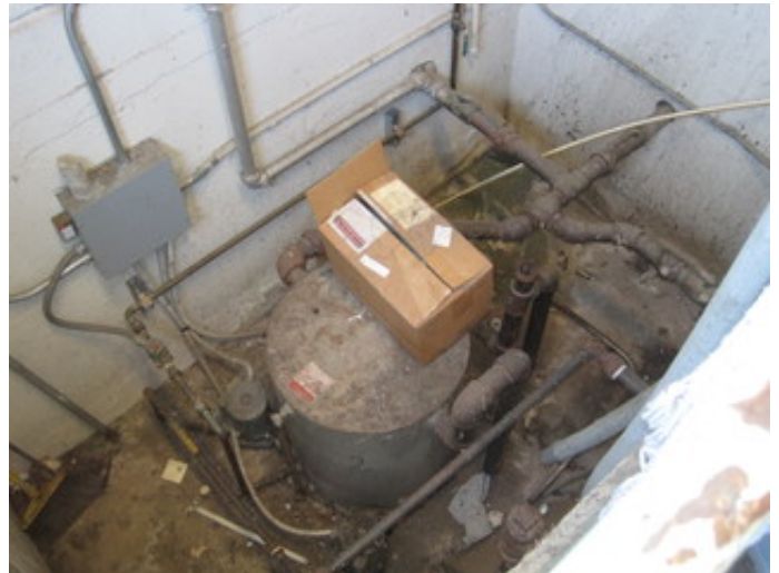
Steam condensate return pump
