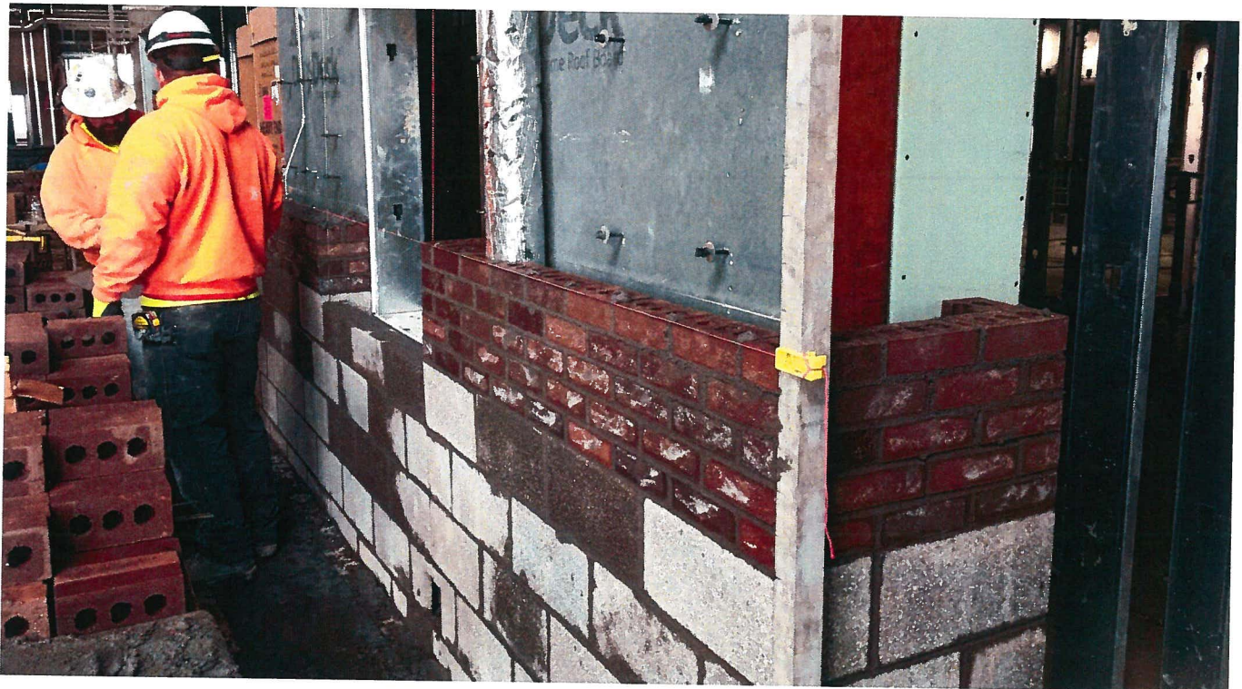
Commons receiving interior brick and masonry at south wall.
