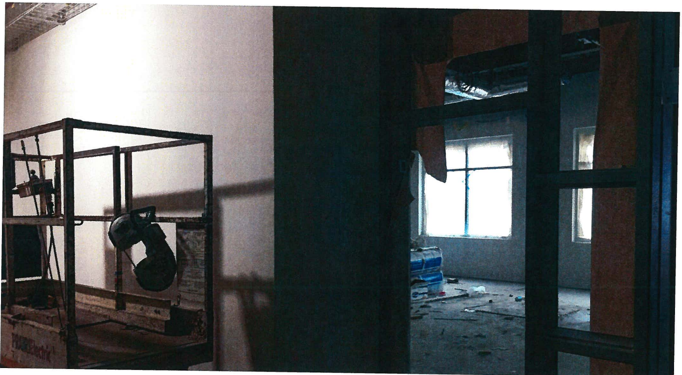
5-6 Wing with paint on interior, glass set, and casework arrives on 3/12.
