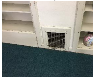
Bathroom Exhaust Grille
