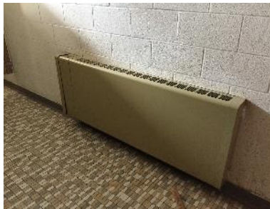
Wall Mounted Radiation
