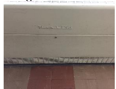
Typical Unit Ventilator
