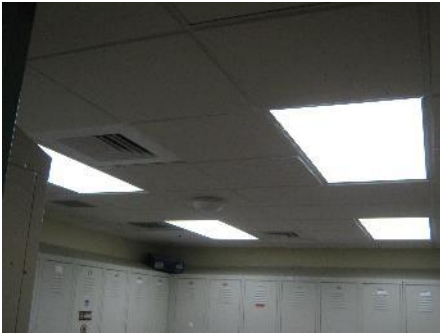
Recessed Lensed Fluorescent Fixture
