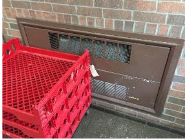
Wall Mounted Radiation
