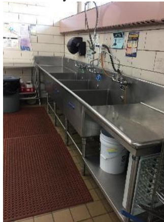
Three Bay Sink in Kitchen
