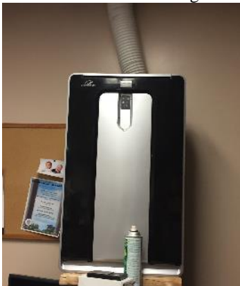
Portable Air Conditioning Unit
