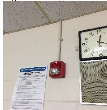
Typical Fire Alarm Horn/Strobe
