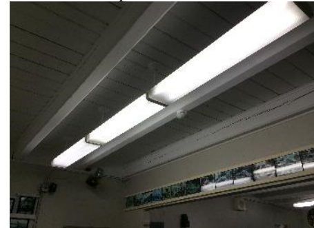
Pendant Mounted Fluorescent Wraparound Fixture
