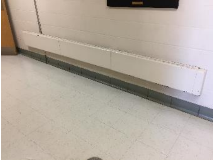
Typical Hot Water Radiation
