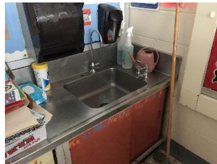
Classroom Sink with Bubbler
