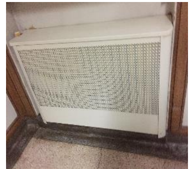
Typical Unit Ventilator
