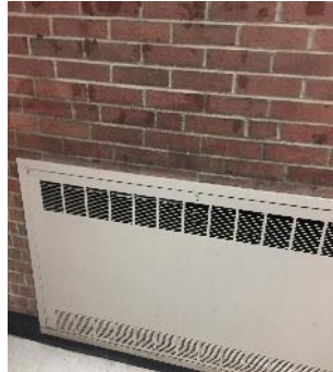
Typical Recessed Wall Mounted Heater
