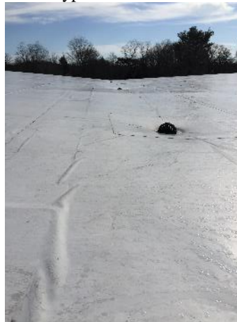
Typical Roof Drain
