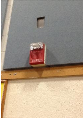
Typical Fire Alarm Horn/Strobe
