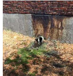
Storm Piping Exiting above Grade
