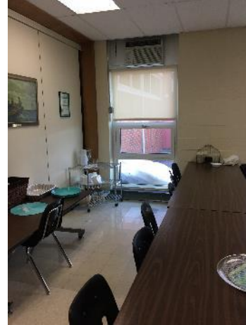
Room with Window A/C Unit
