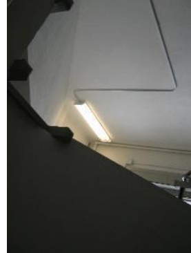
Surface Mounted Wraparound Fixture
