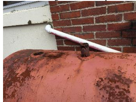
Existing Fuel Tank Top
