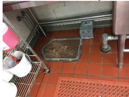
Recessed Grease Interceptor
