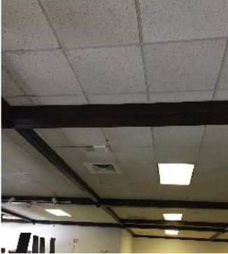
Typical Recessed Fluorescent Fixture
