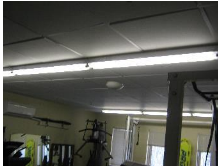
Surface Mounted Fluorescent Fixture
