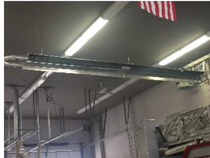
Infrared Heaters
