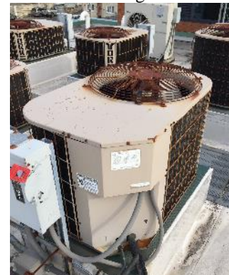
Typical Roof Mounted Condensing Unit
