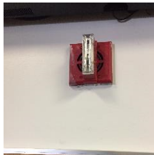
Typical Fire Alarm Horn/Strobe
