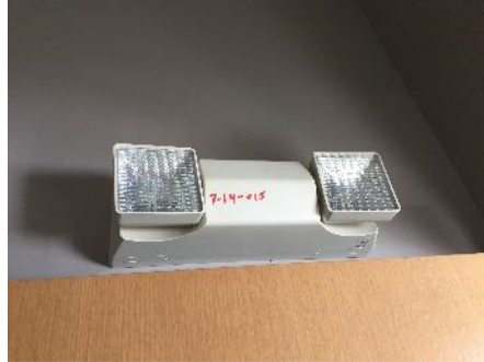
Typical 2-Head Emergency Light Fixture
