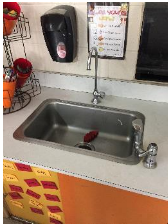
Typical Classroom Sink with Bubbler
