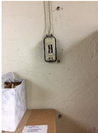
Wall Mounted Thermostat
