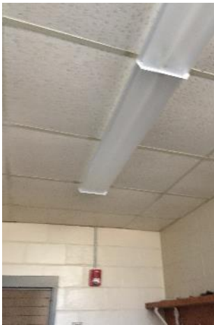
Surface Mounted Fluorescent Wraparound Fixtures
