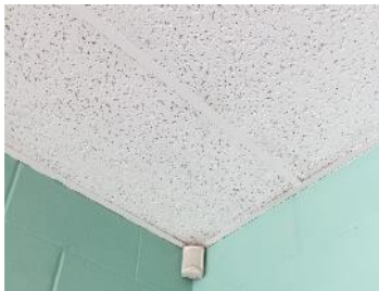
Typical Security System Motion Detector
