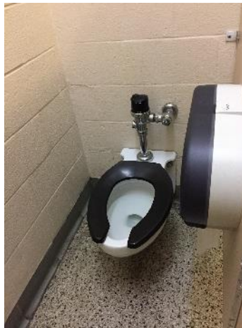
Wall Mounted Water Closet
