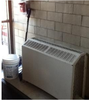
Radiation in Enclosure
