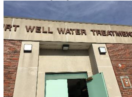
Typical Wall Mounted LED Site Lighting Fixture
