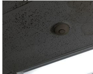
Typical Heat Detector
