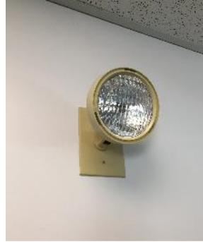
Typical Single Head Emergency Lighting Unit
