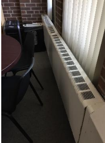
Typical Hot Water Radiation
