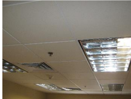
Recessed Parabolic Fluorescent Fixture
