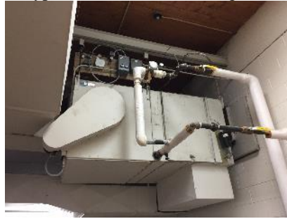
Typical Indoor Air Handling Unit
