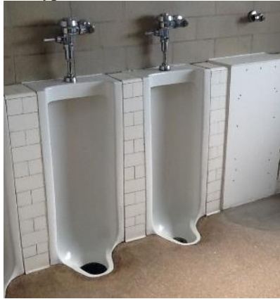
Typical Floor Mounted Urinal
