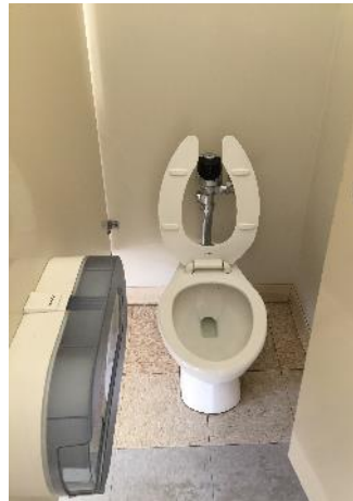
Typical Floor Mounted Water Closet
