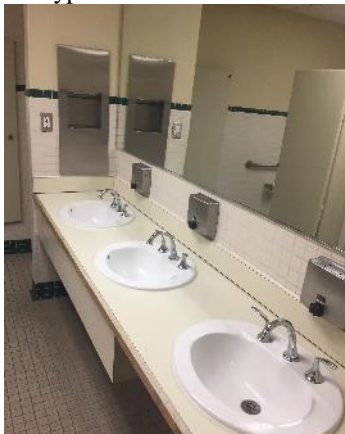
Typical Toilet Room Sink
