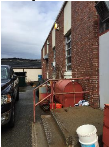
Existing Fuel Tank Location
