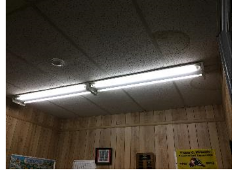
Surface Mounted Fluorescent Fixture
