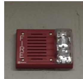
Typical Fire Alarm Horn/Strobe
