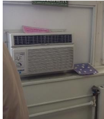
Window Mounted Air Conditioner
