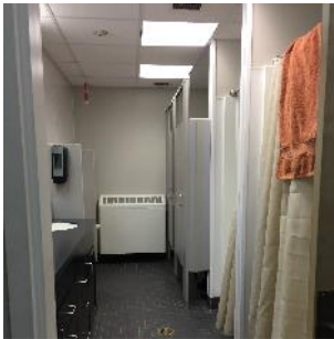
Recessed Fluorescent Fixture
