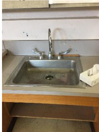
Typical Classroom Sink
