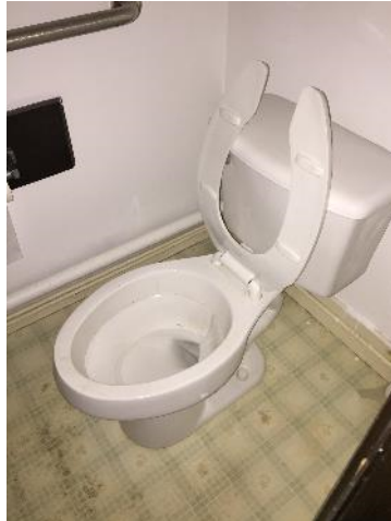
Typical Floor Mounted Water Closet
