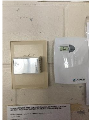
Wall Mounted Thermostat
