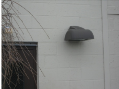
Wall mounted Full Cut-off Fixture
