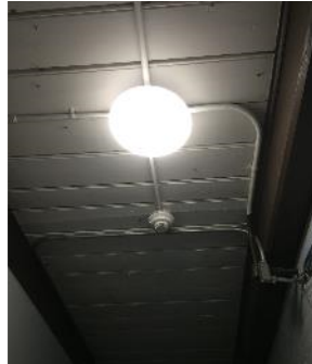
Surface Mounted Fixture
