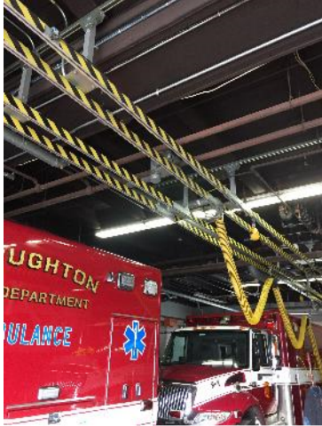
Plymovent Vehicle Exhaust System
