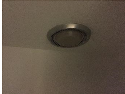
Toilet Exhaust Fan with Light
