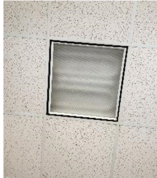
Typical Recessed Fluorescent Fixture
