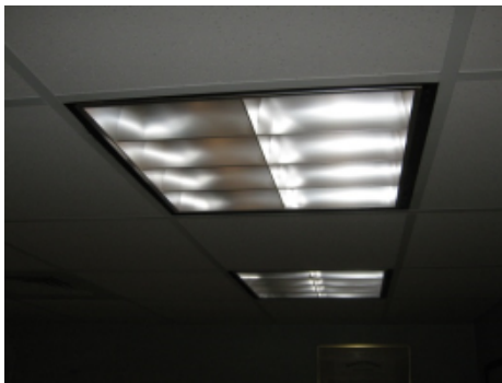
Recessed Parabolic Lighting Fixture
