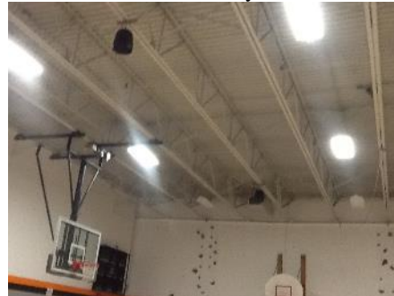
Surface Mounted Fluorescent Wraparound Fixture
