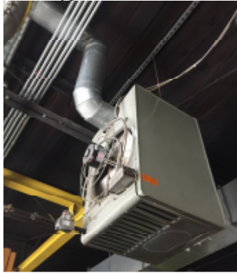
Typical Unit Heater
