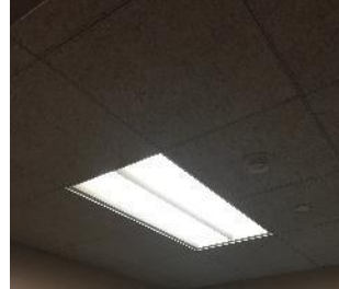
Typical Recessed Fluorescent Fixture
