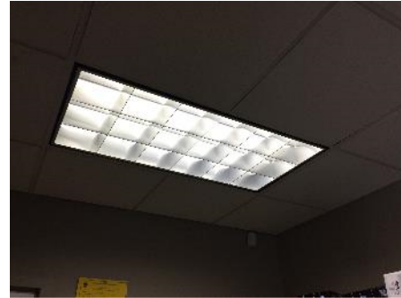
Recessed Parabolic Fixture
