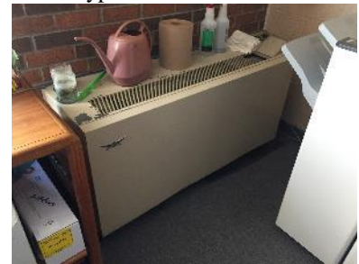
Typical Unit Ventilator
