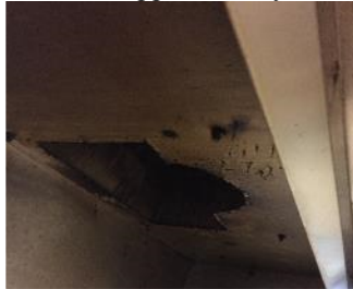
Kitchen Hood with no Filters or Fire Suppression System
