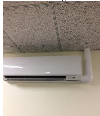
VRF System Wall Mounted Air Handling Unit
