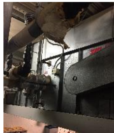
Typical Air Handling Unit
