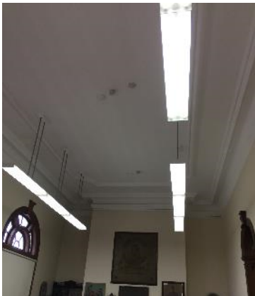
Pendant Mounted Wraparound Fluorescent Fixtures
