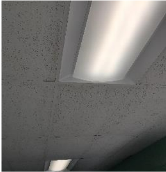
Typical Recessed Fluorescent Fixture
