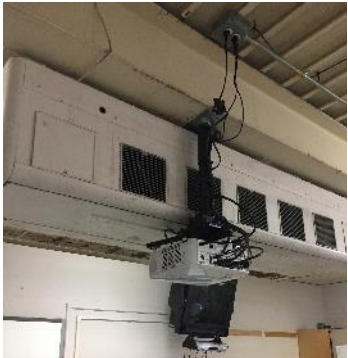
Typical Ceiling Mounted Unit Ventilator
