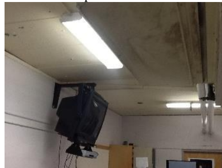
Surface Mounted Fluorescent Wraparound Fixture
