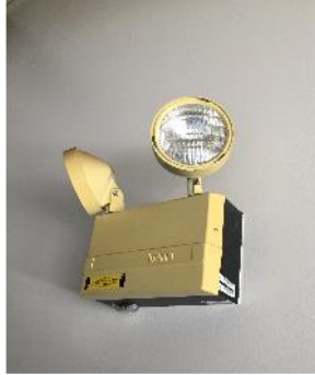
Typical 2-Head Emergency Lighting Unit
