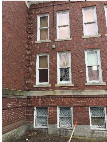
Wall Mounted Site Lighting Fixture
