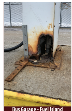
Bus Garage - Fuel Island
