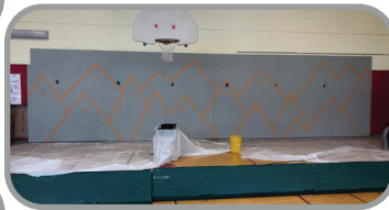
A work in progress
