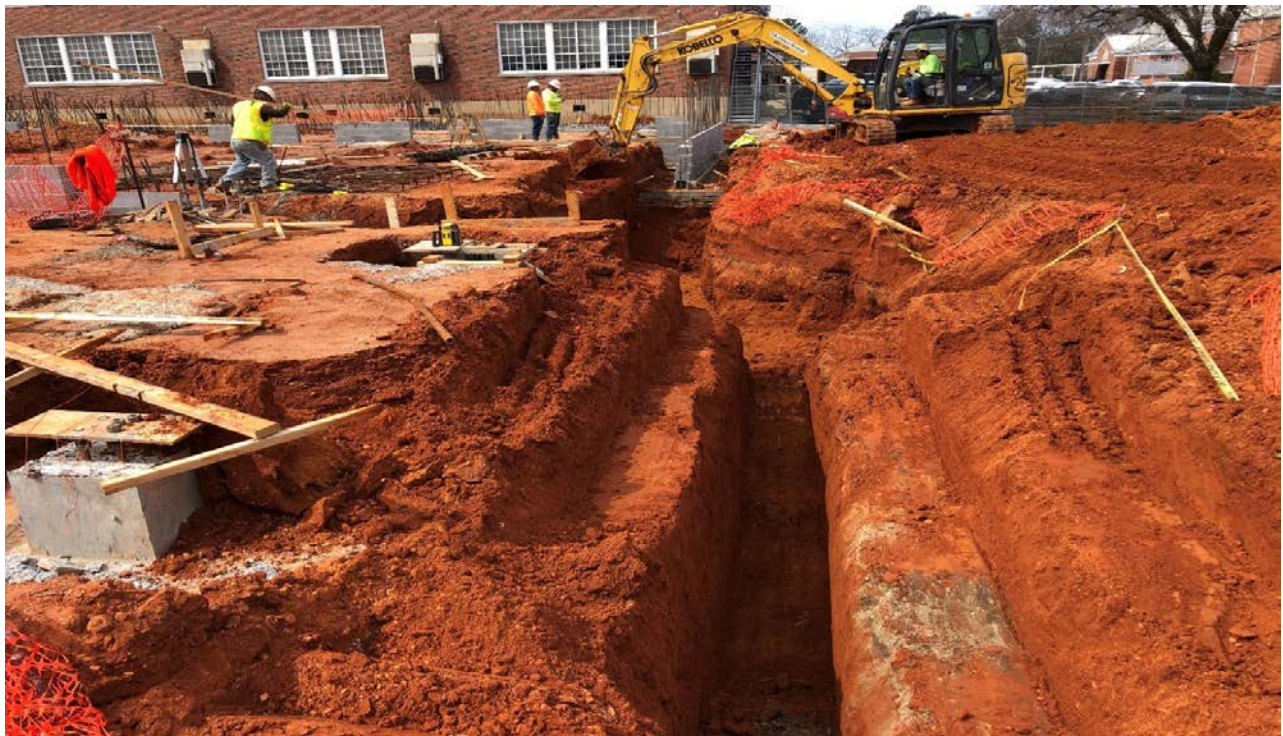
Cleaning out footings after rain on 03-05-2021
