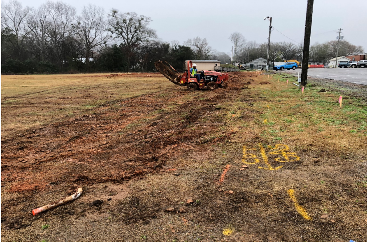
Underground conduits for portable classrooms on 02-11-2021
