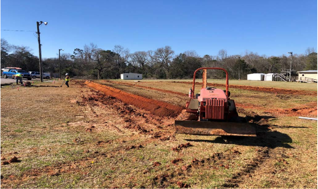
Underground conduits for portable classrooms on 02-19-2021
