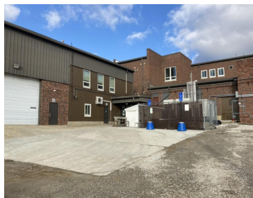
West Door View #2
