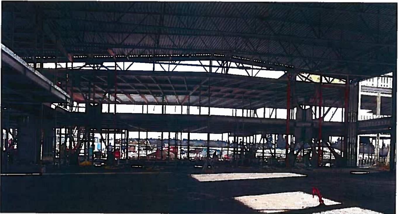
Cafeteria area with roof deck in place
