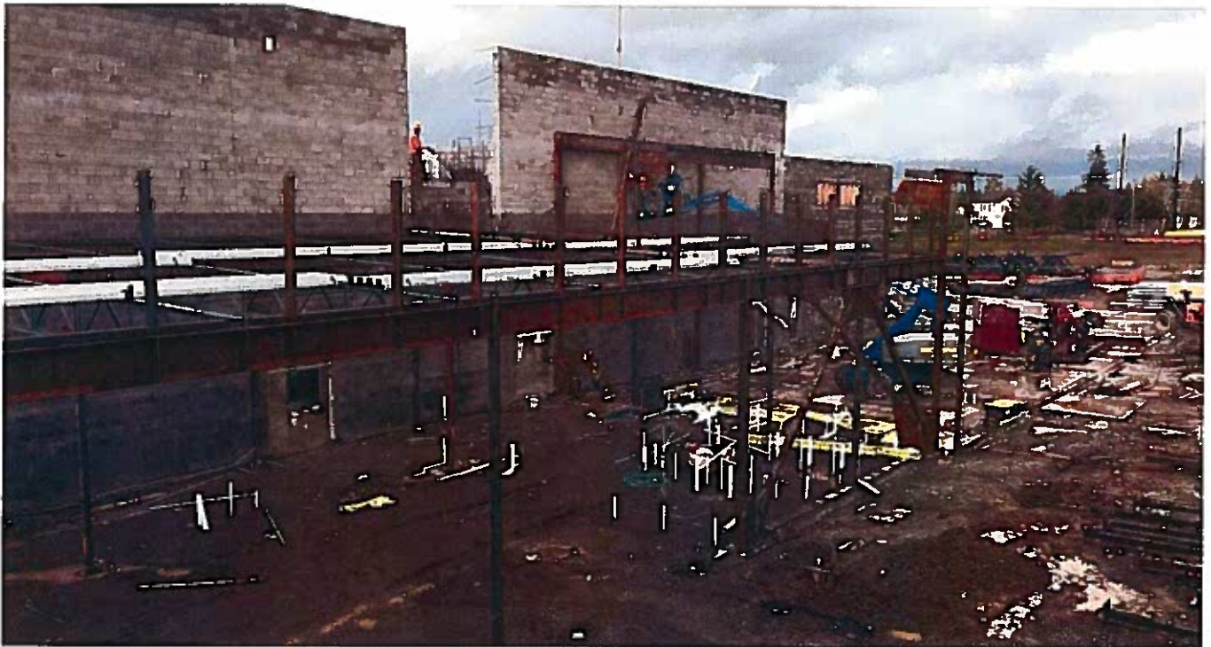
Last month of steel going up now – here at locker rooms
