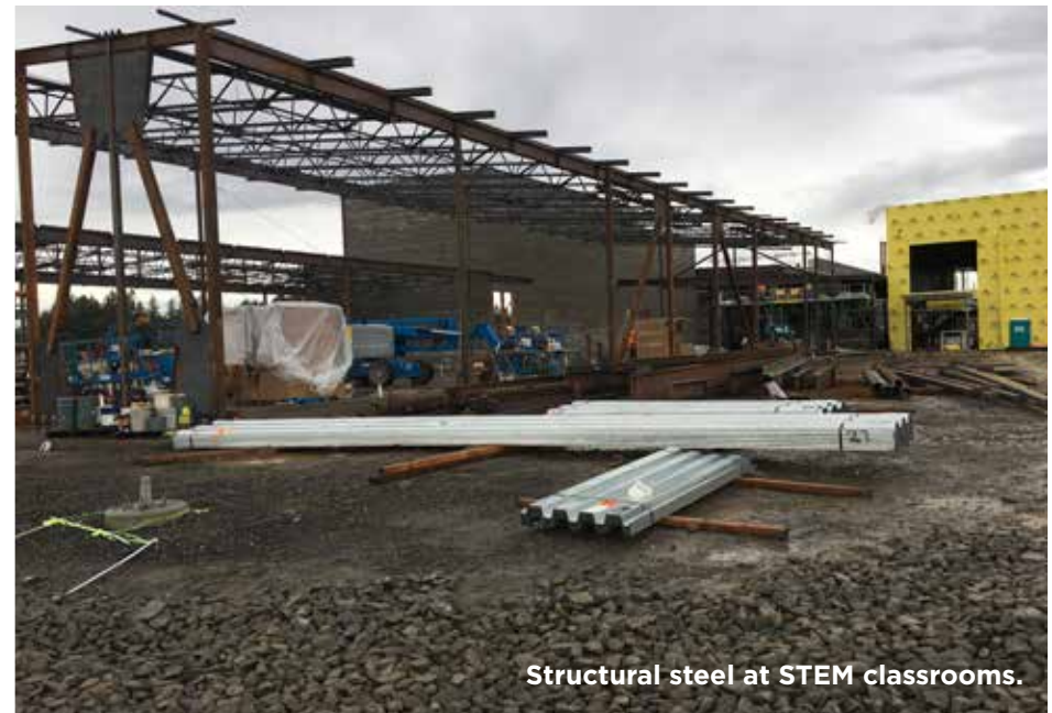
At far left, structural steel work in progress in 7/8 classroom wing while work on exterior wall framing continues in 5/6 classroom wing (at right).
