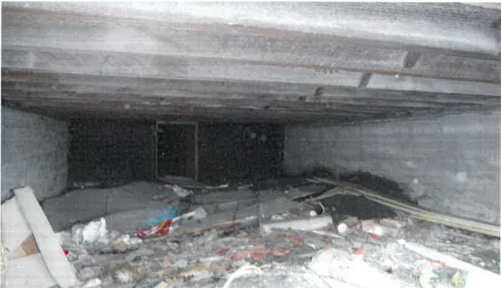
Typical Crawlspace and Floor Framing
