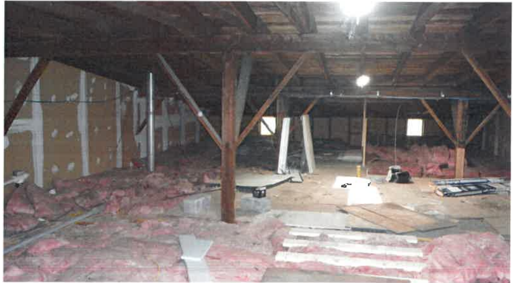
Attic, No Storage, Access Only
