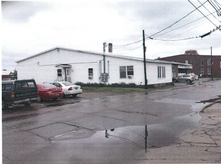
26-30 Catherine Street, South East View
