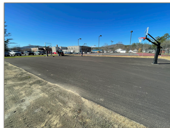
The outdoor basketball court at DHS nearing its completion!
